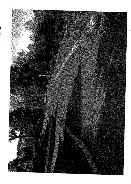
2" Thick - 3/8" Clean Stone Wearing Surface 6" Thick Recycled Concrete Aggregate (RCA) Base Course
